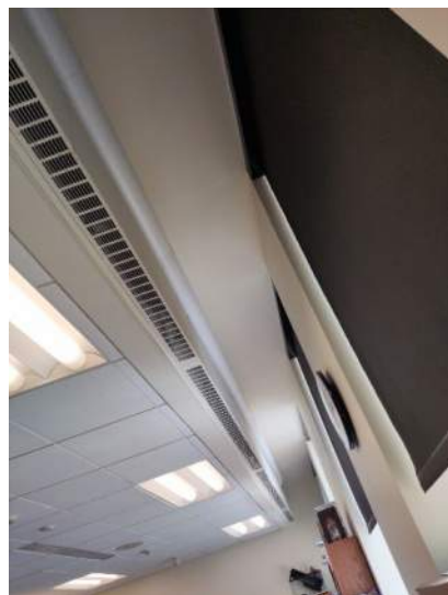
FIN TUBE HEATING AT PERIMETER
