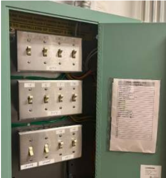
EXAMPLE OF RELAY PANEL CONVERSION
