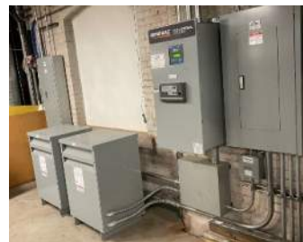
ATS AND DISTRIBUTION ARRANGEMENT
