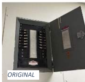
TYPICAL BRANCH CIRCUIT PANELS
